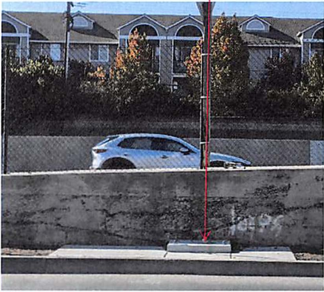
TOLLING ITEM #2: FOUNDATION PAD FOR MODEL 332L CABINET FOR VARIABLE TOLL MESSAGE SIGN
